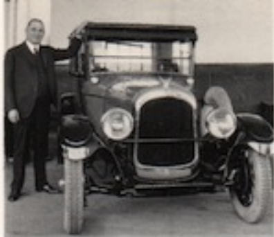
Walter P. Chrysler next to his 1924 namesake, which came with an L-head six — the first high-compression production engine.
