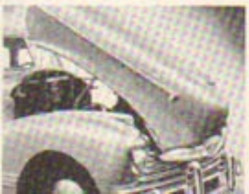
Safest hood design—hinged at the front and locked from inside.
