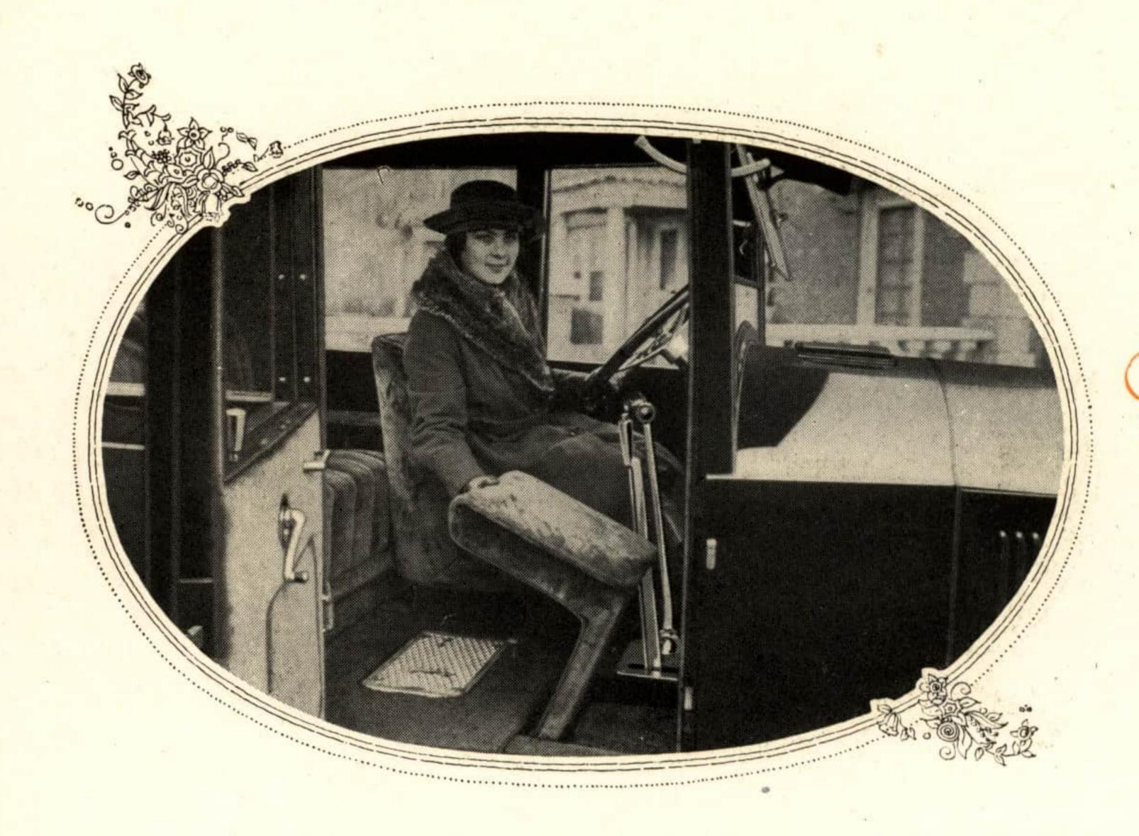
he ease with which the auxiliary chair is lifted into position, and its substantial construction are shown here. Noteworthy also is the scientifically correct position of the driver's seat—levers close at hand so that they may be operated without change of posture
