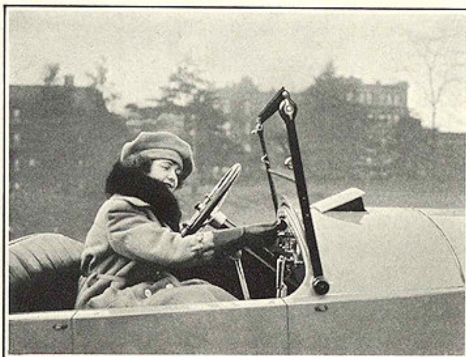
Ventilator is easily and quickly adjusted from dash
