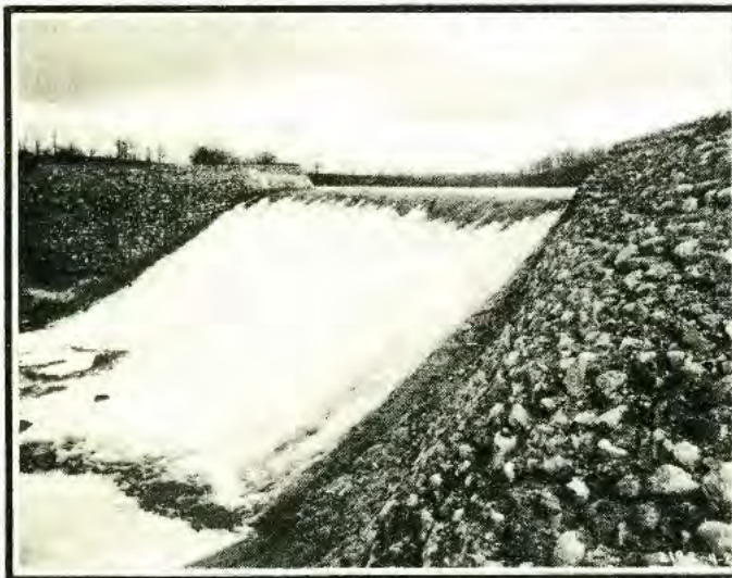
Water coming over the dam at Phoenix, Mich.
