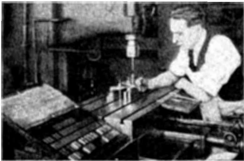
Milling a fixture with the aid of Ford-Johansson gages
