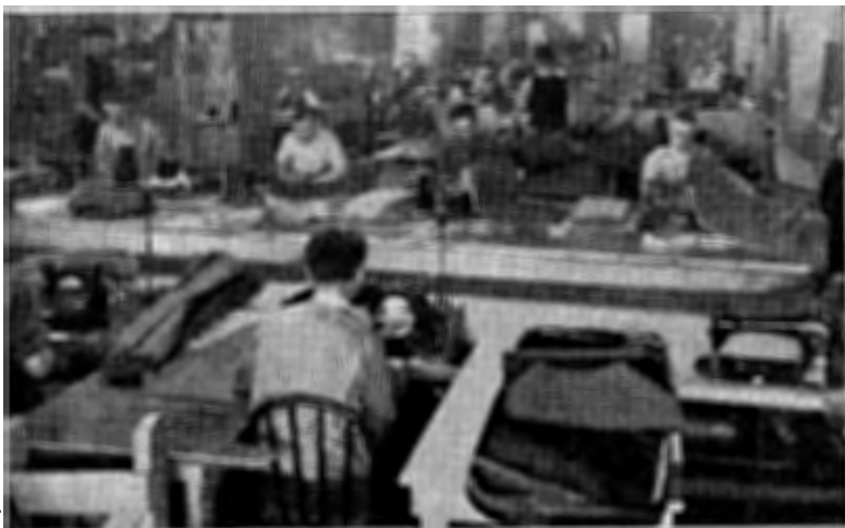
Scene in the upholstery department at the Highland Park plant
