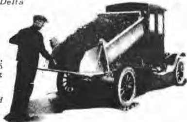
View of body hoisted, with apron plates No. 3006 adjusted for easy shoveling of coal.
