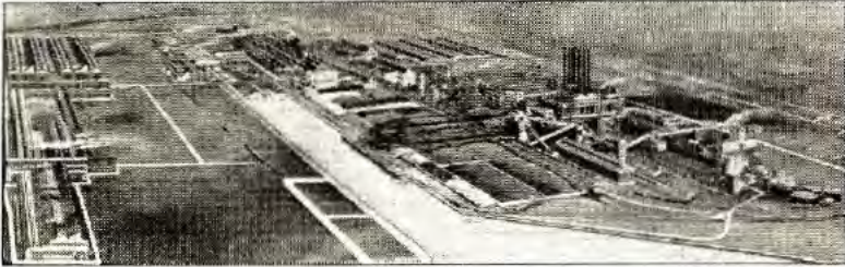
The Fordson Plant
