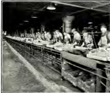
Each Radiator Tested For Leaks
