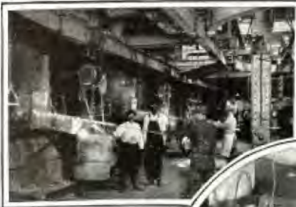
Filling a Ladle at a Cupola.
