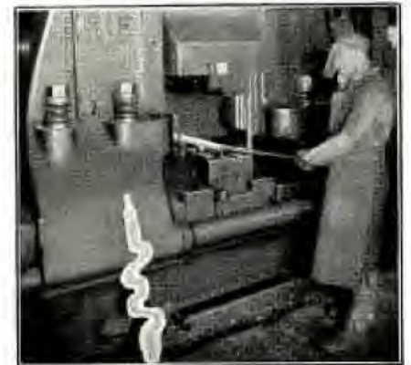
Steam Hammer Forges Crankshafts
