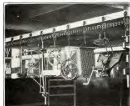
THE FORD CONVEYOR SYSTEM Above and below you see Conveyors at work, bringing parts and materials to the men who stand still at their work. This departure from previous practice saves both time and the energy of the workmen.
