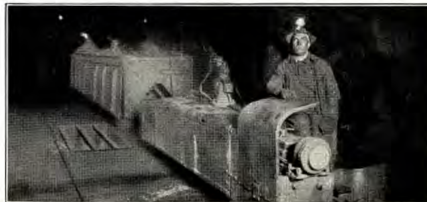
A Trainload of Ore Being Dumped into the Skip.
