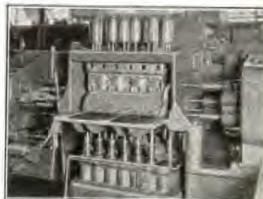
Boring 48 Holes at a Single Operation
