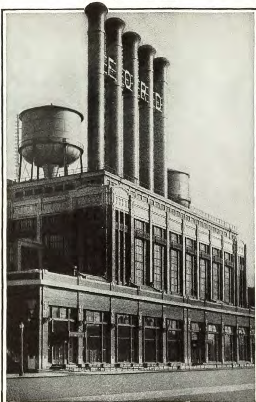
THE HIGHLAND PARK POWER HOUSE
