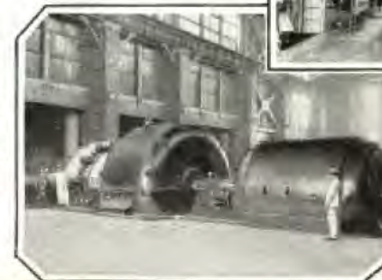
The Furnace Room. Left: 62,500 H. P. Turbo Generator
