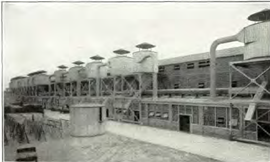
A Building Where Wood Working is Carried On.—Note the Dust Collectors to Keep the Air Clean.
