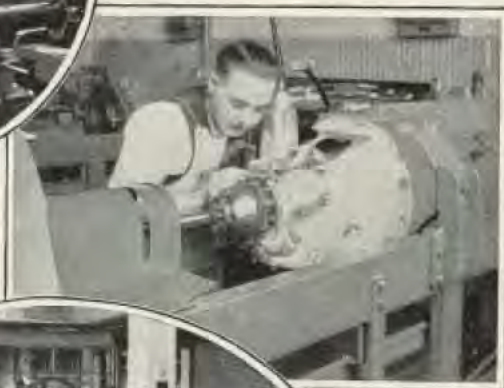
Testing Gears in the "Quiet Room"
