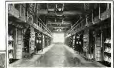
The Furnace Room. Left: 62,500 H. P. Turbo Generator
