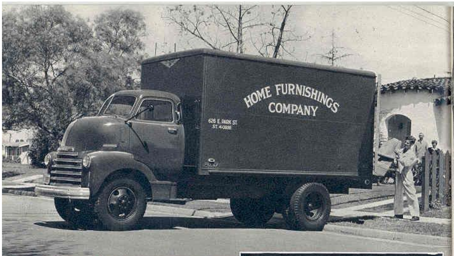
MODEL 3703 CHASSIS AND CAB 155-INCH WHEELBASE, MAXIMUM G.V.W., 16,000 LB.
