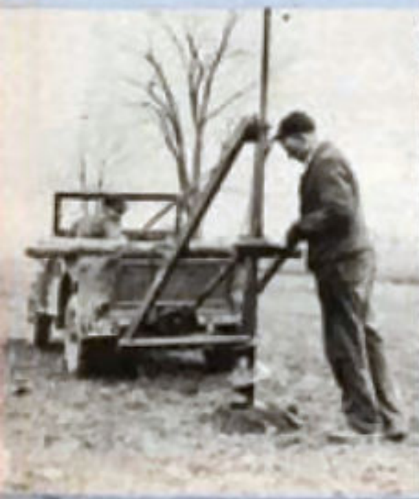
10" power-driven post hole auger
