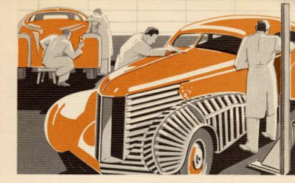
Through the preliminary stages of design development miniature scale models provide a ready means of translating the idea and sketches of the artist into three-dimensional form. But later, when the new design approaches its final stages, full-size models must be made in order to be certain that the design is entirely harmonious.
