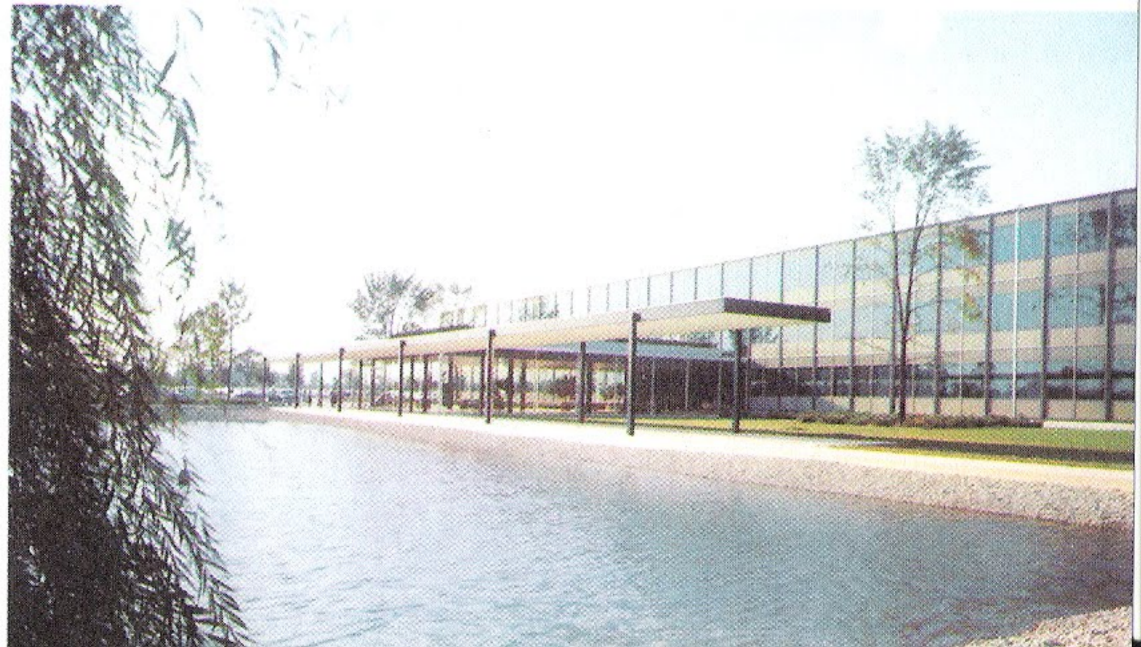
South facade of Research Building.
