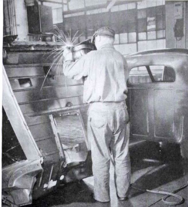
Top, back, and bottom sections of truck cab are gas-welded into single unit in former passenger car body plant.
