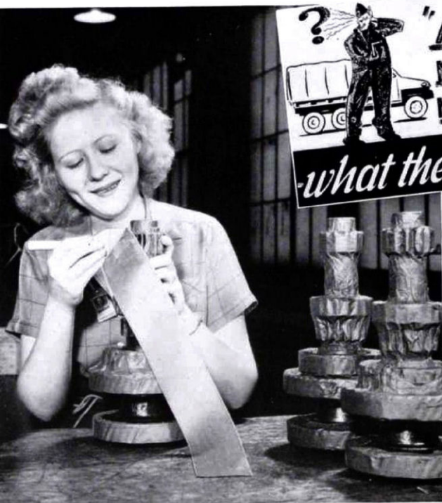
"Mold wrapping" a cluster gear reveals how carefully truck parts are protected against rust and corrosion for shipment overseas.
